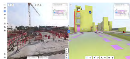
Design verification can be performed by comparing 360 degrees image of actual site and BIM model Image Courtesy of CLP Power Hong Kong Limited
