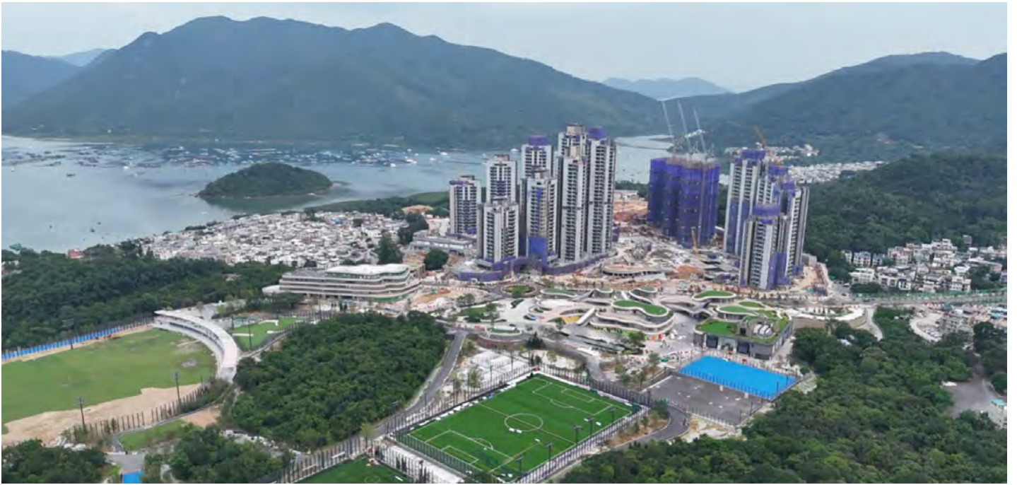
Site aerial image Image Courtesy of Sun Hung Kai Properties Limited and Sanfield (Management) Limited and Strategic Building Innovation (SBI) bimSCORE Limited
