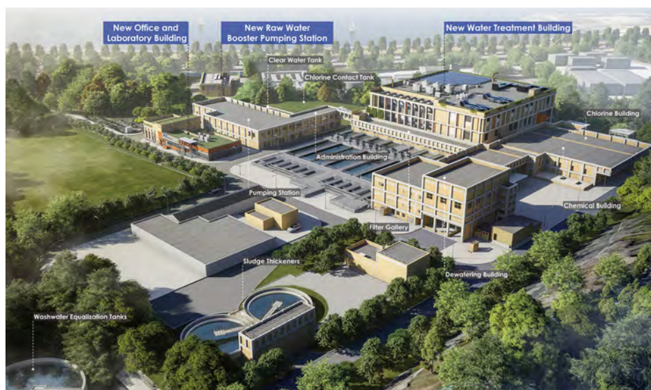
Works Completion Renderings of SHWWTW Extension Works Image Courtesy of Water Supplies Department, HKSAR Government and China Road and Bridge Corporation and Digie Engineering Technology Pte. Ltd.
