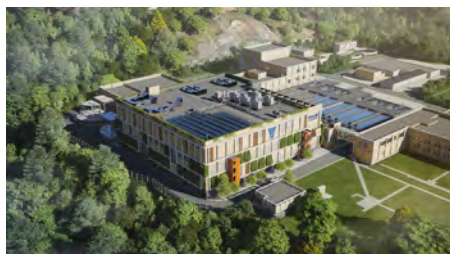
New Water Treatment Works Building Image Courtesy of Water Supplies Department, HKSAR Government and China Road and Bridge Corporation and Digie Engineering Technology Pte. Ltd.
