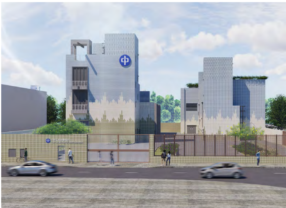
CLP Power's Yuen Long Industrial Estate Substation Image Courtesy of CLP Power Hong Kong Limited
