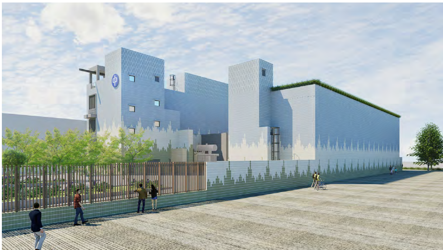
CLP Power's Yuen Long Industrial Estate Substation achieved our aim to integrating sustainable development principles and design thinking through BIM technologies Image Courtesy of CLP Power Hong Kong Limited
