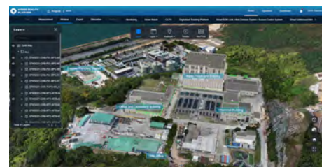
Hybrid Reality Centralized Management Platform Image Courtesy of Water Supplies Department, HKSAR Government and China Road and Bridge Corporation and Digie Engineering Technology Pte. Ltd.
