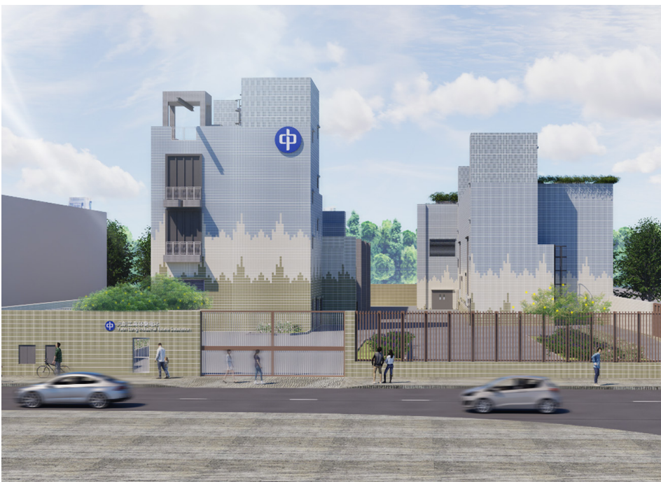
CLP Power's Yuen Long Industrial Estate Substation Image Courtesy of CLP Power Hong Kong Limited
