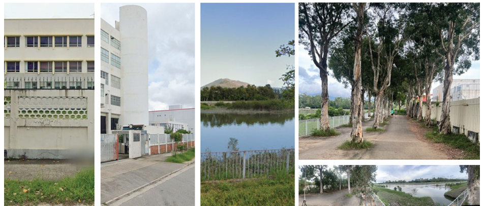
Natural landscape of Nam Sang Wai and the industrial building in Yuen Long Industrial Estate Image Courtesy of CLP Power Hong Kong Limited
