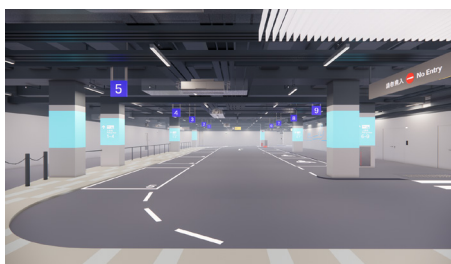
Automated Carpark A Lay-by Area Rendering Image Courtesy of Paul Y. - CIMC - JEC Joint Venture
