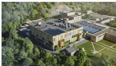
New Water Treatment Works Building Image Courtesy of Water Supplies Department, HKSAR Government and China Road and Bridge Corporation and Digie Engineering Technology Pte. Ltd.
