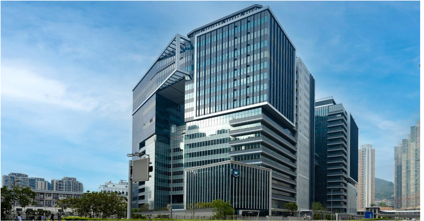
Immigration Headquarters Overview Image Courtesy of Architectural Services Department, HKSAR and Hip Hing Engineering Company Limited
