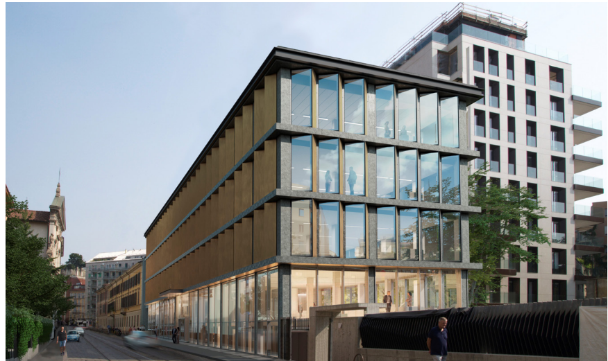
The project team retained the existing structure, fully reconstructing the interiors and adding a new facade.
