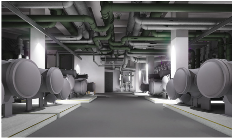
3D BIM Simulation of DCS Plant Image Courtesy of CRBC-QH-REC-QTEC Joint Venture and Binnies Hong Kong Limited and Huadong Engineering (Shenzhen) Corporation Limited
