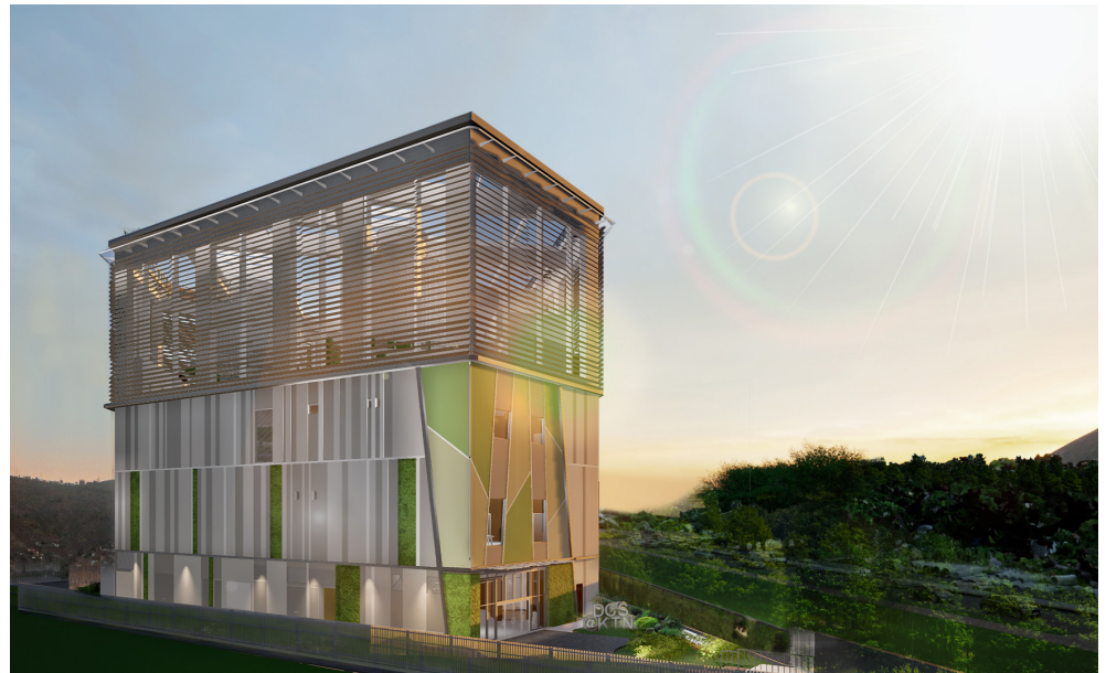
Overall View of the Phase 1 District Cooling System at Kwu Tung North New Development Area Image Courtesy of CRBC-QH-REC-QTEC Joint Venture and Binnies Hong Kong Limited and Huadong Engineering (Shenzhen) Corporation Limited
