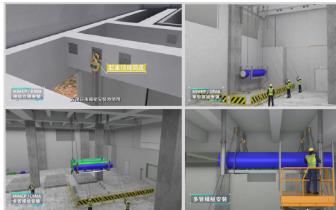
Installation Simulation for DfMA Image Courtesy of CRBC-QH-REC-QTEC Joint Venture and Binnies Hong Kong Limited and Huadong Engineering (Shenzhen) Corporation Limited
