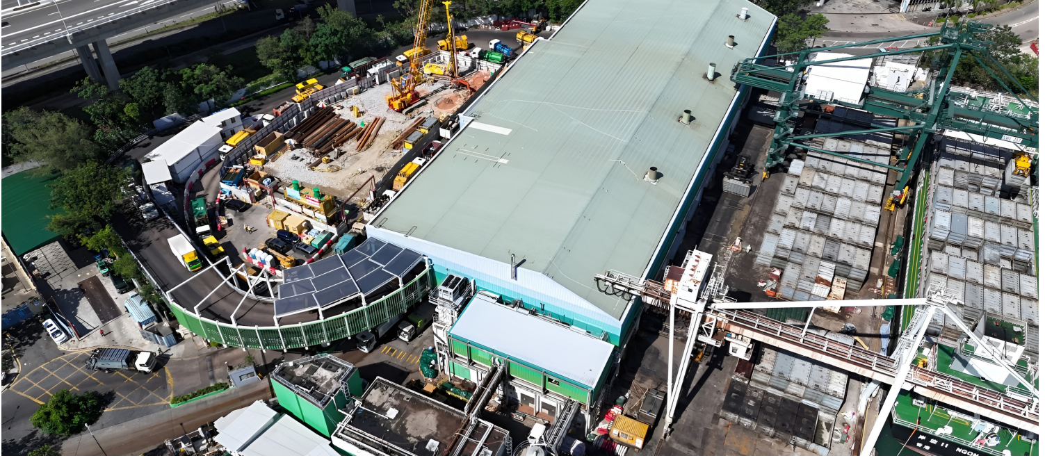
Overview of WKTS Image Courtesy of Environmental Protection Department, the Government of the Hong Kong Special Administrative Region & AECOM Asia Company Limited & China Harbour Engineering Company Limited
