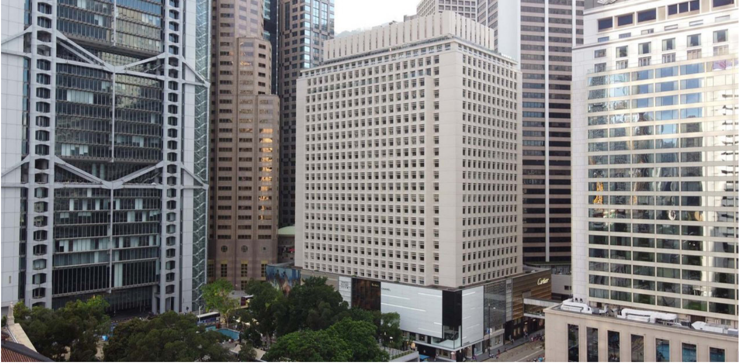
Prince's Building Image Courtesy Hongkong Land Limited and Gammon Construction Limited
