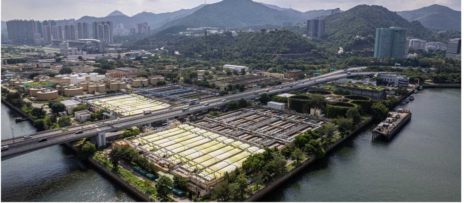
Existing Sewage Treatment Works Image Courtesy of Drainage Services Department, the Government of the Hong Kong Special Administrative Region and AECOM Asia Company Limited and China State Construction Engineering (Hong Kong) Limited – Alchmex International Construction Limited Joint Venture
