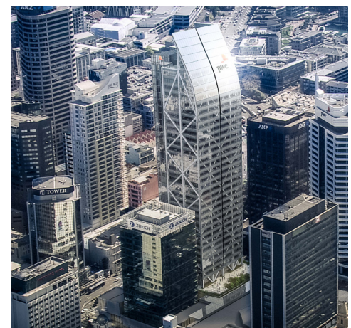
Image courtesy of Warren and Mahoney: Commercial Bay in association with Woods Bagot and NH Architecture.
