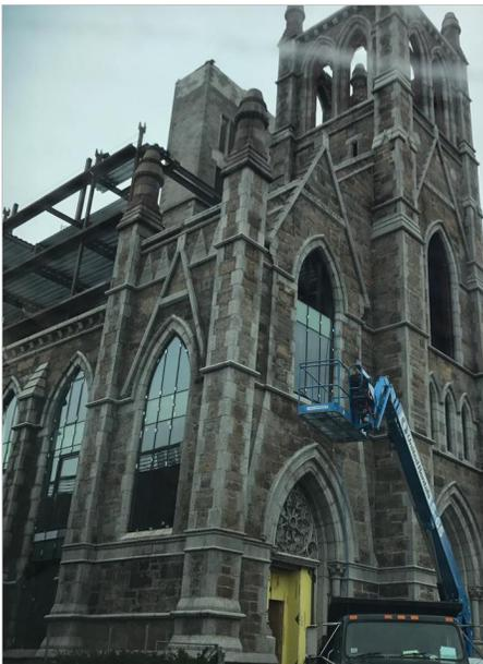
Several years ago, Lawton Welding, a miscellaneous metals and small structural steel company based in Topsfield, Massachusetts, took on a project detailing and fabricating the steelwork for an old stone church that was being renovated and repurposed. The project was fraught with rework orders – largely due to the irregularities of the stone structure – and took nearly three months to complete.
