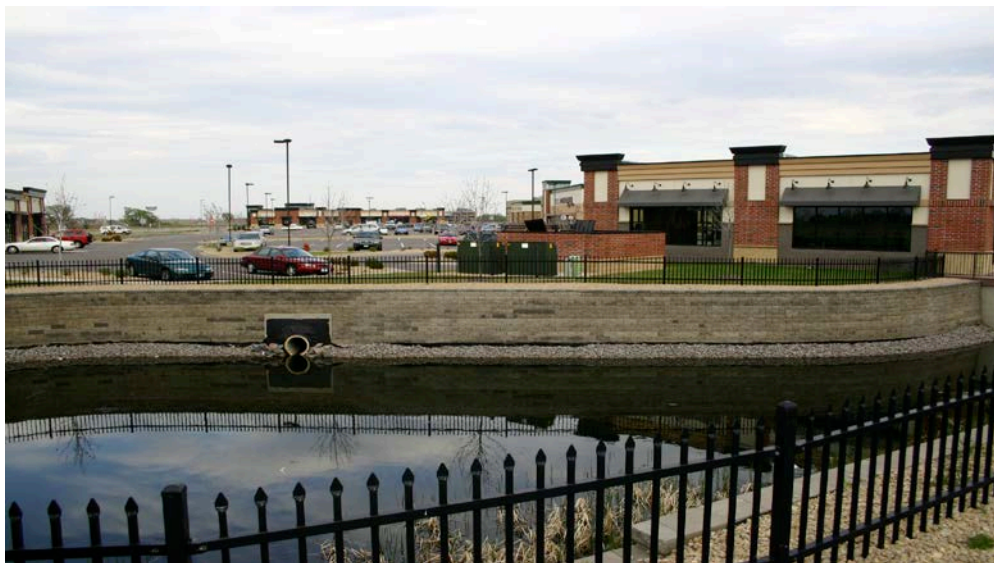
Typical commercial detention basin and development in Ramsey. Image courtesy of Bolton & Menk, Inc.
