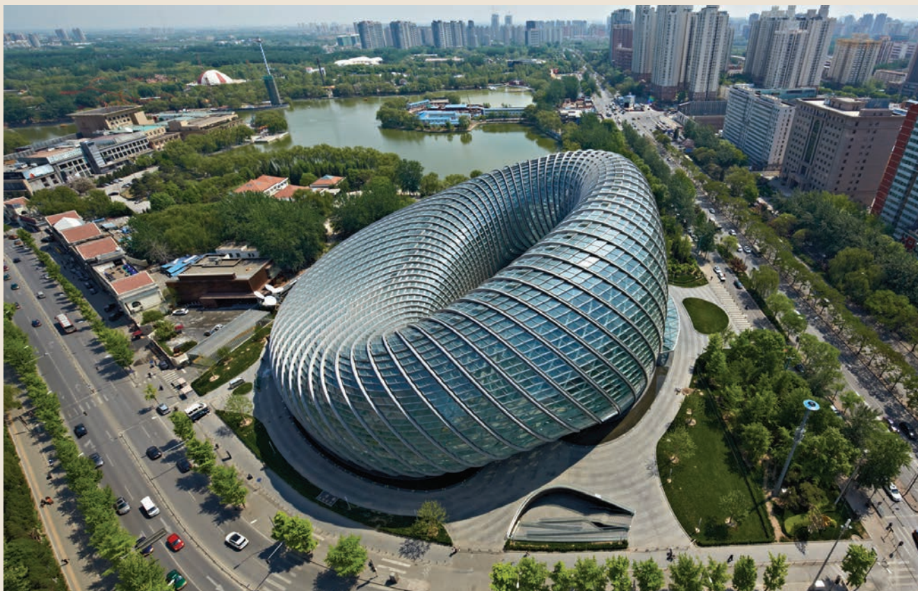
The striking torus shape of the Phoenix Media Center was made possible by the use of BIM by the design team.
