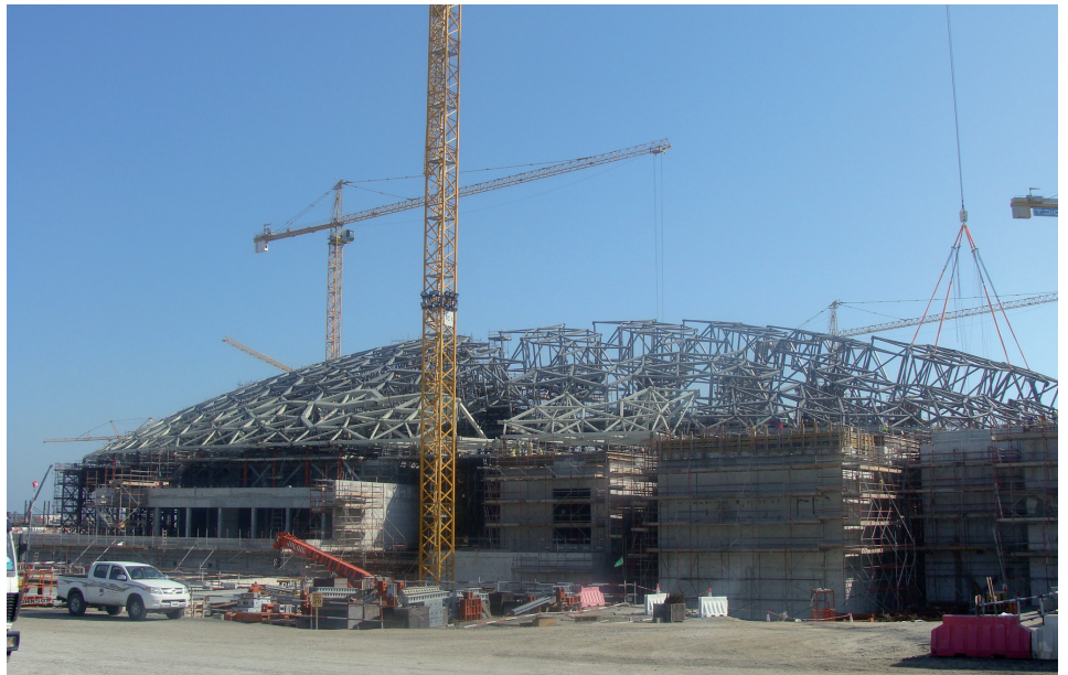
Dome under construction (Image courtesy of Waagner-Biro)
