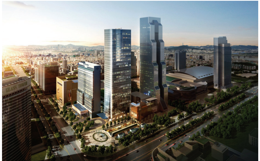
Aerial view of the Parnas Tower
